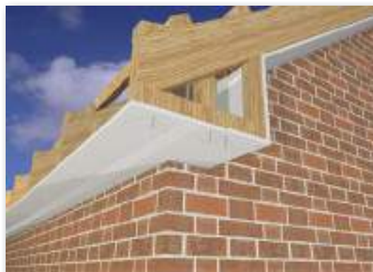
Fig 9. Typical GPBV soffit installation.
