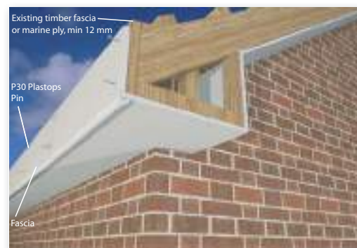
Fig. 17. Standard over-fascia installation.
