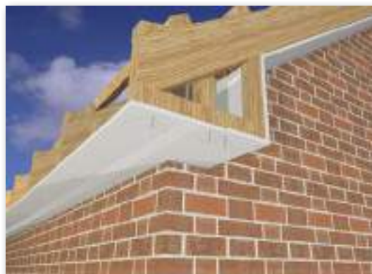
Fig 20a. Typical GPBV soffit installation.
